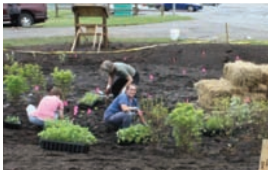
Above: Longswamp Township, Berks County, demonstration rain garden. Signage explains that that rain gardens are designed to absorb and filter off pollutants carried by stormwater.
